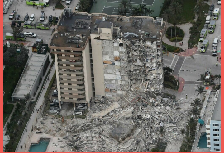
The tragic collapse of a condominium building in Surfside, Florida last year has triggered a wave of legislation to update regulations for condos. Photo via Florida Politics..
